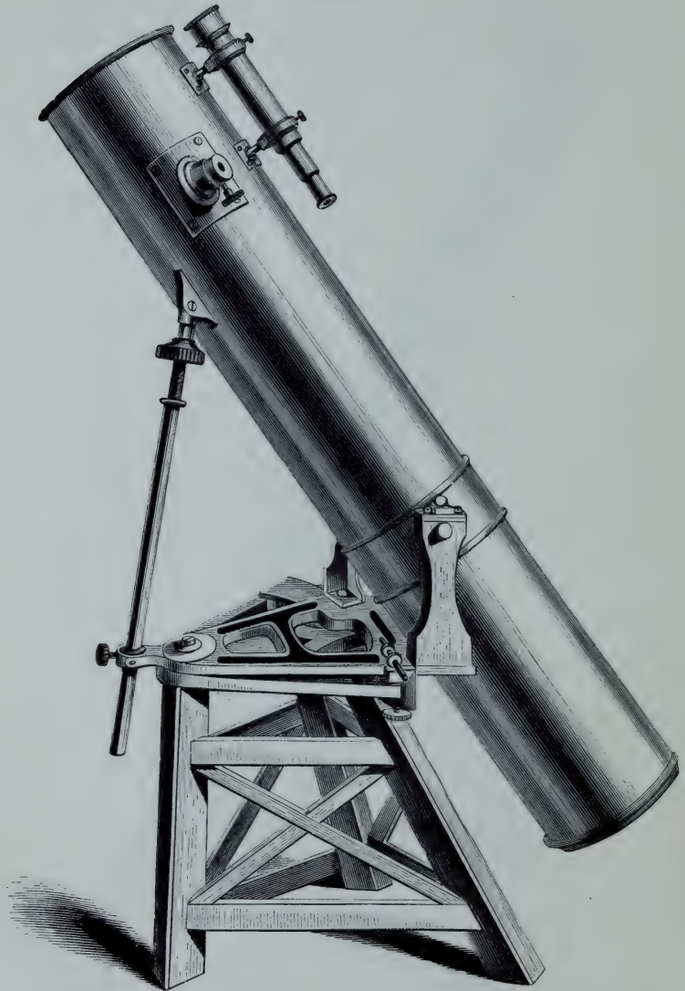
ALTAZIMUTH MOUNTING FOR A LARGE REFLECTOR. ( By Browning. )
